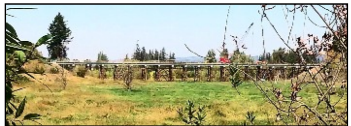
Looking north towards the Onion Flats area of the Tonquin Floods Channels. The train trestle reveals the depth of the channel itself
