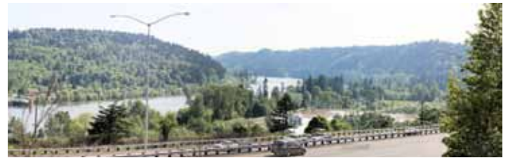
Figure 3. Oregon City Gap from the north
